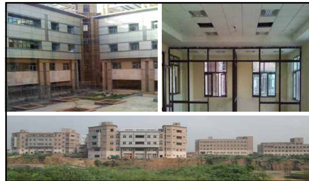
Construction at Faridabad site
